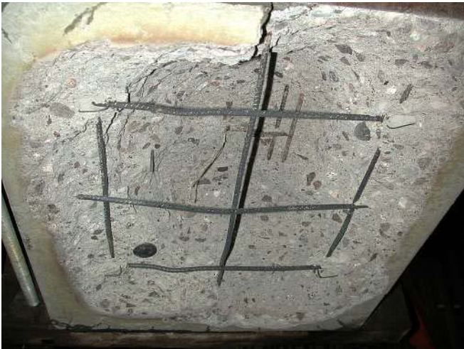
Figure E23. Small slab SS 40 03 after the fire test.
