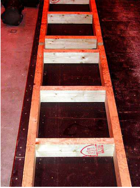
Figure F9. Mould for small slabs.
