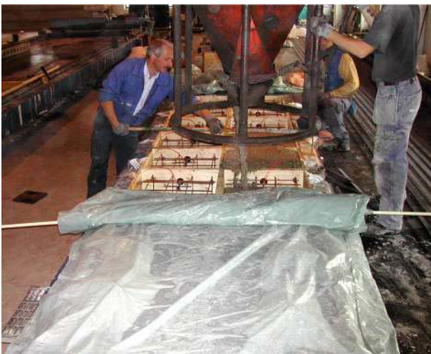
Figure D5. Casting of large slabs and protection with plastic foil.
