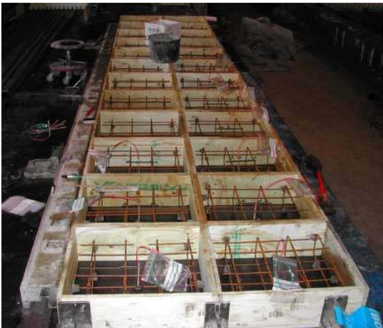
Figure E6. Casting moulds and reinforcement for small slabs.
