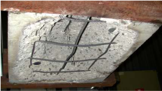
Figure E25. Small slab SS 40 04 after the fire test.
