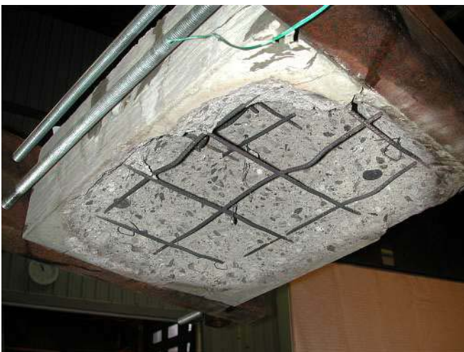
Figure E17. Small slab SS 30 04 after the fire test.
