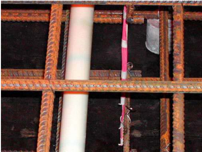
Figure F2. Mounting of thermocouples in a large slab.
