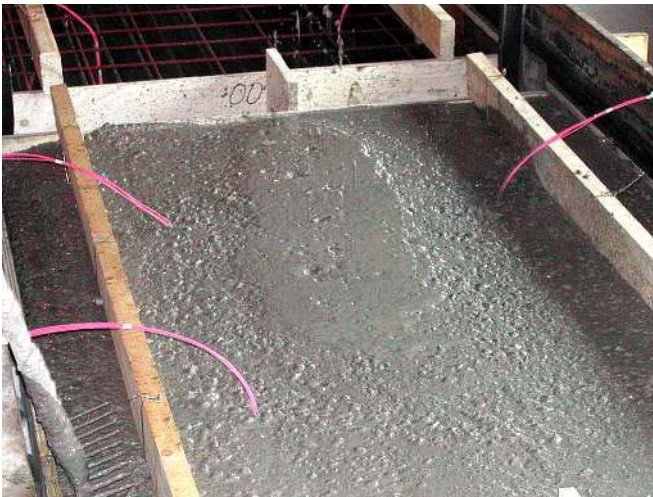
Figure D4. Casting of large slabs.
