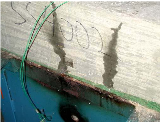
Figure E20. Small slab SS 40 02 during the fire test. Water is pouring out at the edges.
