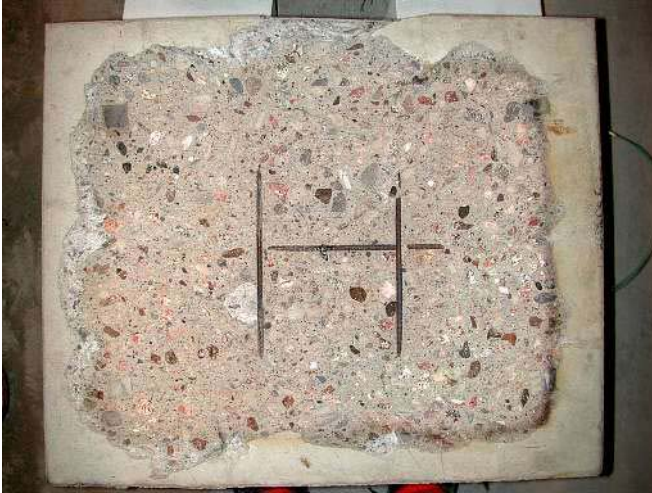
Figure E21. Small slab SS 40 02 after the fire test.
