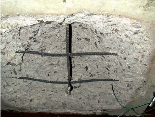
Figure E36. Small slab SS 55 04 after the fire test.
