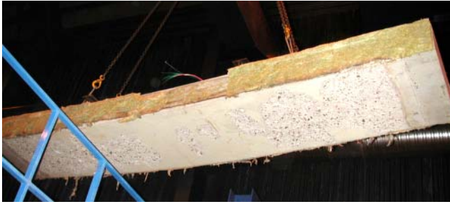
Figure D15. Beam LB 40 01 after the fire test.
