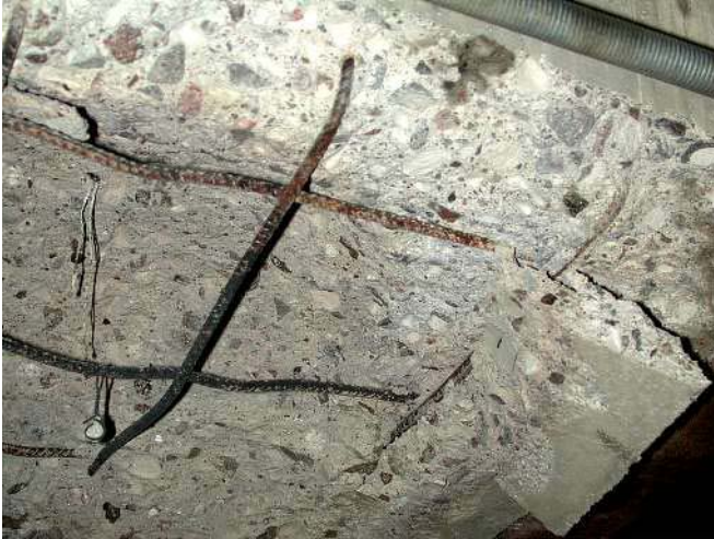
Figure E35. Close-up on small slab SS 55 03 after the fire test.
