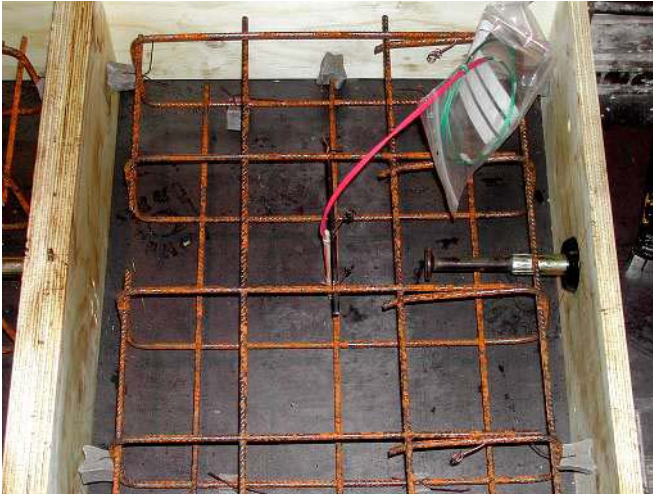
Figure E5. Casting mould and reinforcement of small slabs.
