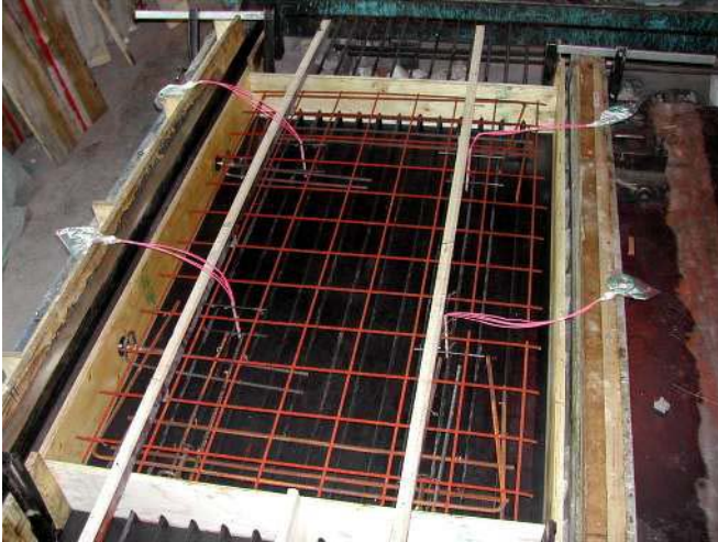
Figure D3. Reinforcement of large slabs.
