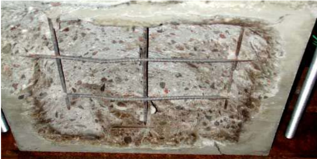
Figure E15. Small slab SS 30 03 after the fire test.
