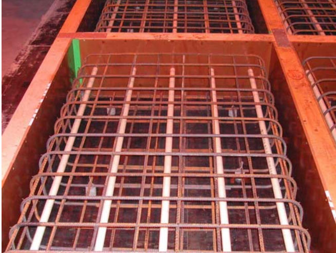
Figure F1. Reinforcement of large slabs.
